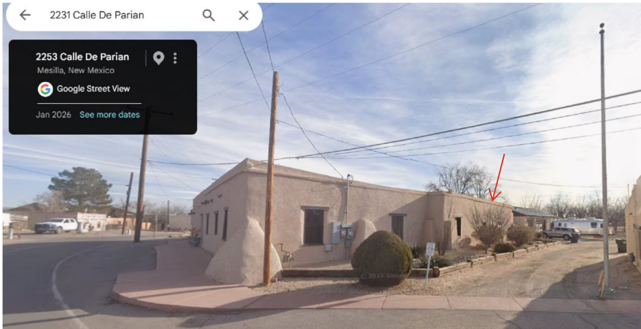
Requested new A/C unit installation area
