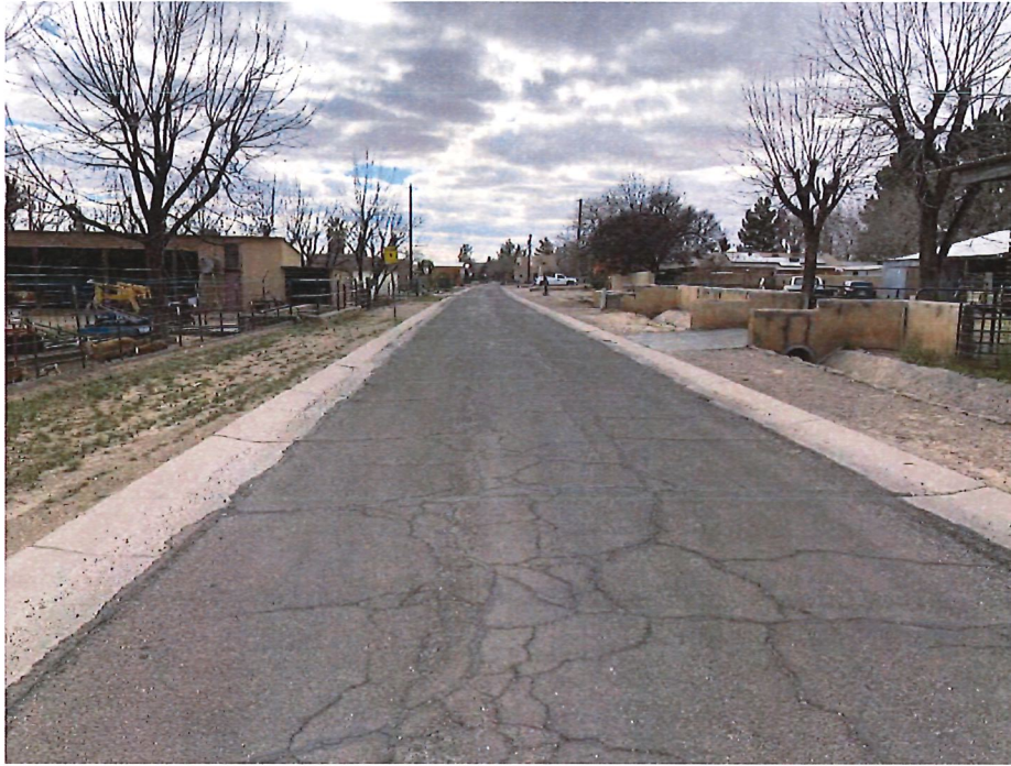
Photo 1. Calle de Colon – Current Road Conditions - West view near Calle Primera
