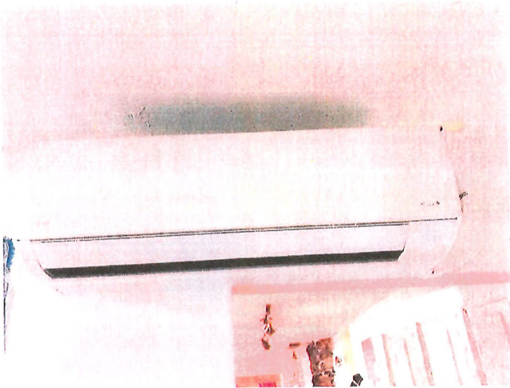
Air conditioning rewiring in the kitchen
