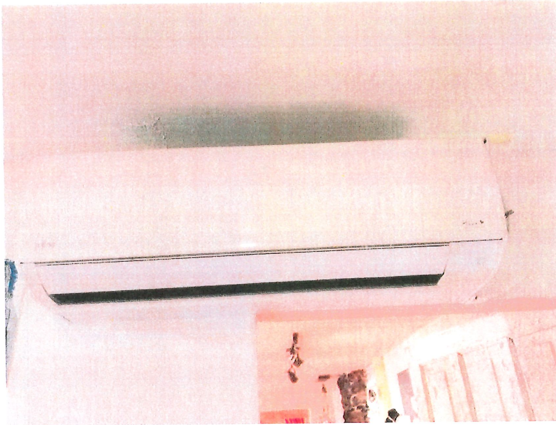
Air conditioning rewiring in the kitchen
