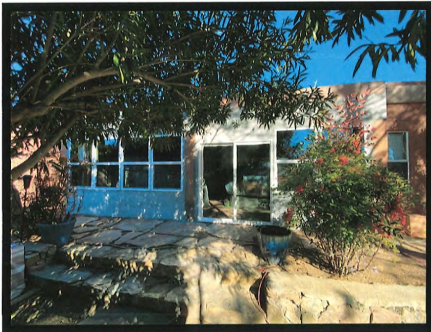
Elevation of new construction
