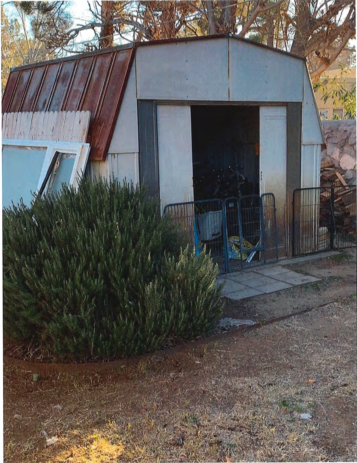
Existing (original?) utility shed to be removed
