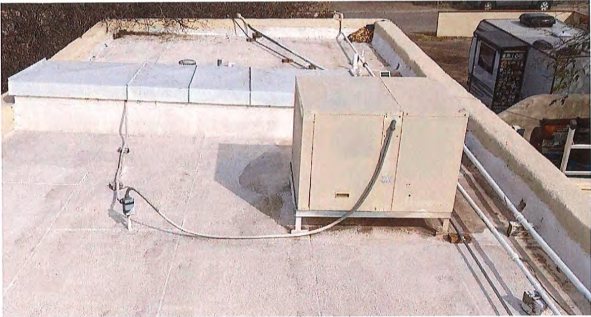
Picture of the Existing Evaporative Cooler and Metal Box Containing the Furnace
