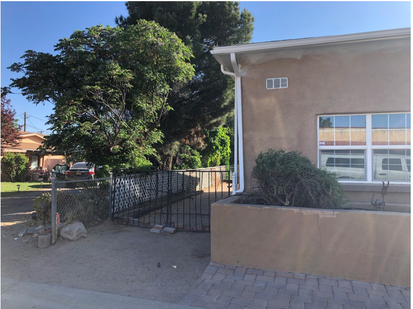
Above Photo: Existing Gate at northwest side of home. New Gate will be located in same location; New Gate will be split at center and swing in both directions as Existing Gate.
