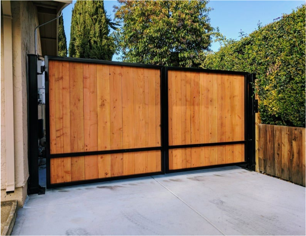
GATE DESIGN/STYLE - Above image shows similar example of alternate metal frame and cedar panel gate design/style/construction.
