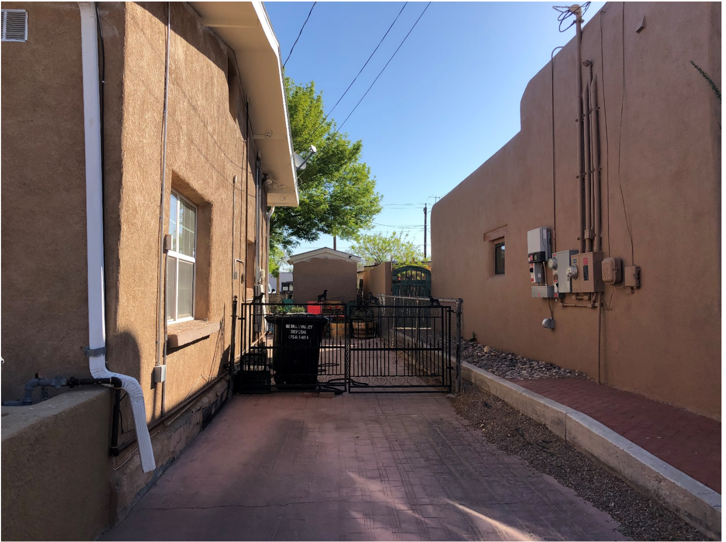
Above Photo: Existing Gate at southwest side of home. New Gate will be located in same location; New Gate will be split at center and swing in both directions as Existing Gate.
