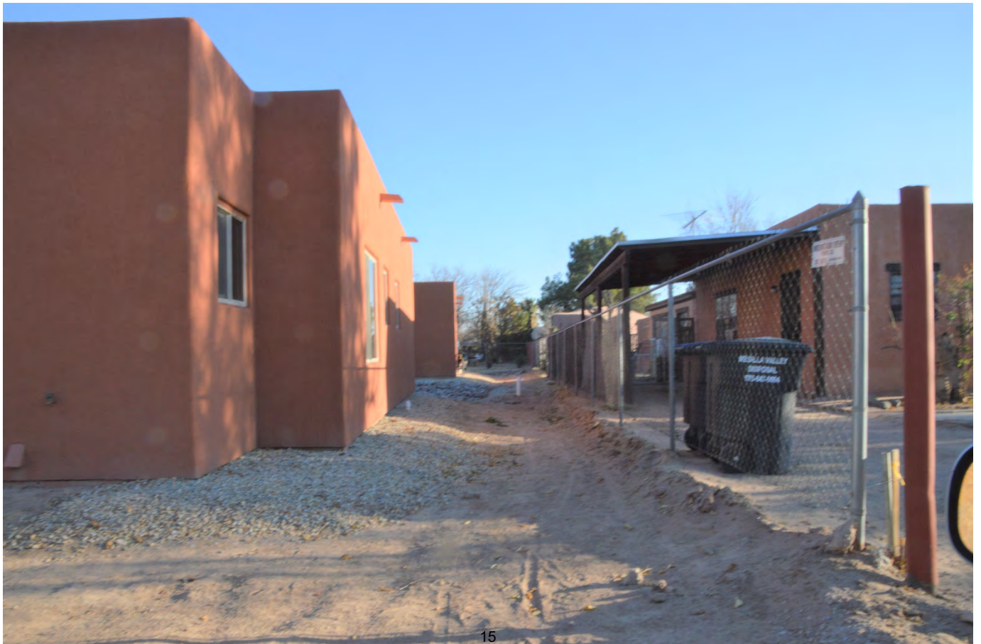
PHOTO SHOWING THE REAR OF THE PROPERTY FROM CALLE DE COLON
