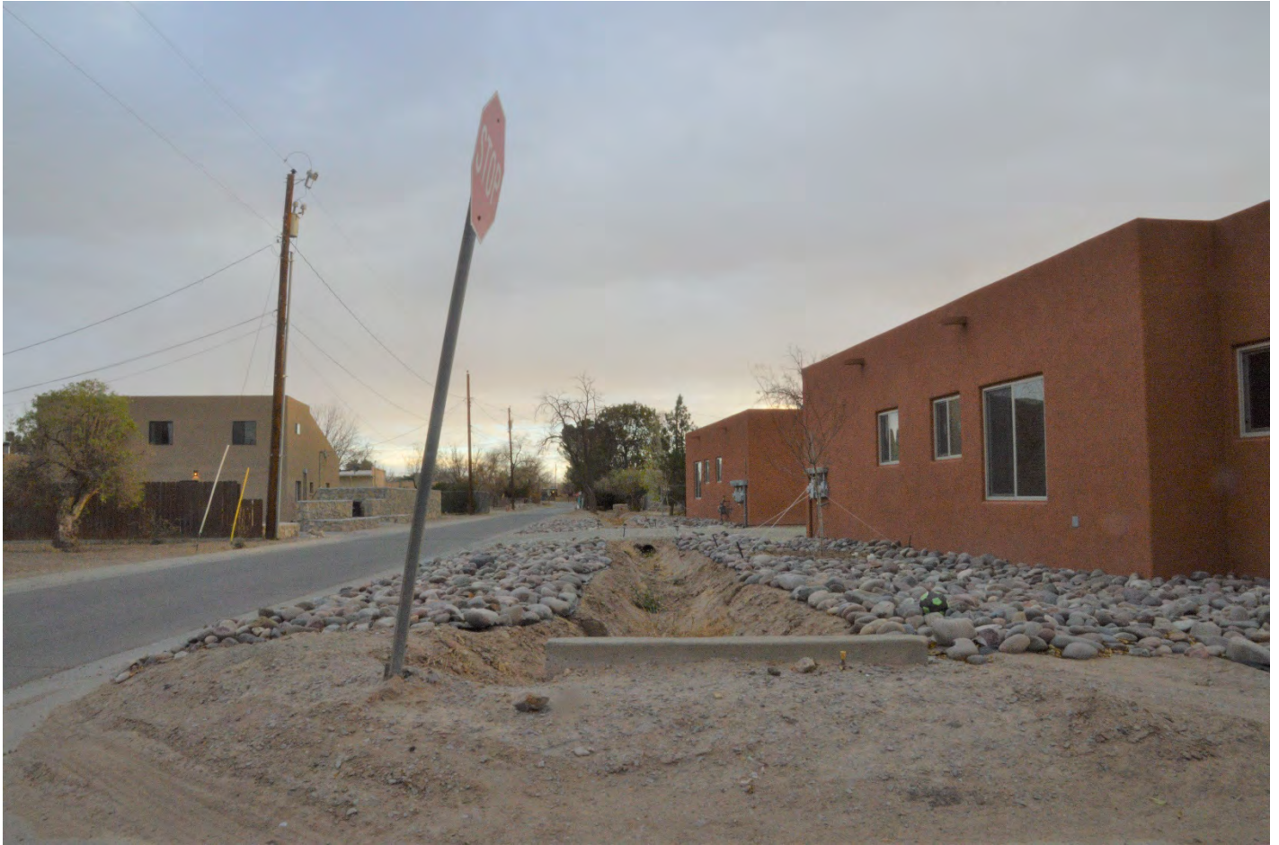
PHOTO OF THE PROPERTY FROM CALLE TERCERA
