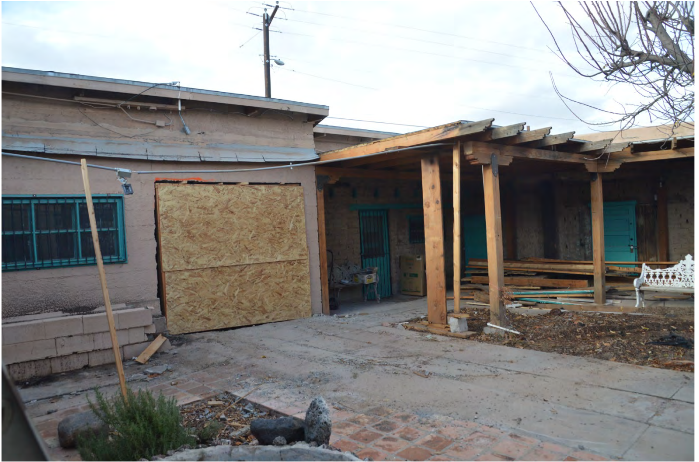
PHOTO OF REAR OF DWELLING SHOWING EXTERIOR WORK (Taken 12/27/18)
