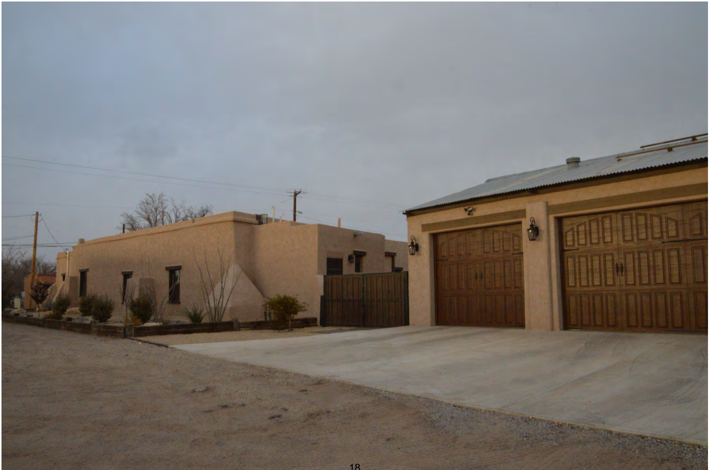
PHOTO OF THE DWELLING FROM THE POST OFFICE SHOWING THE GARAGE
