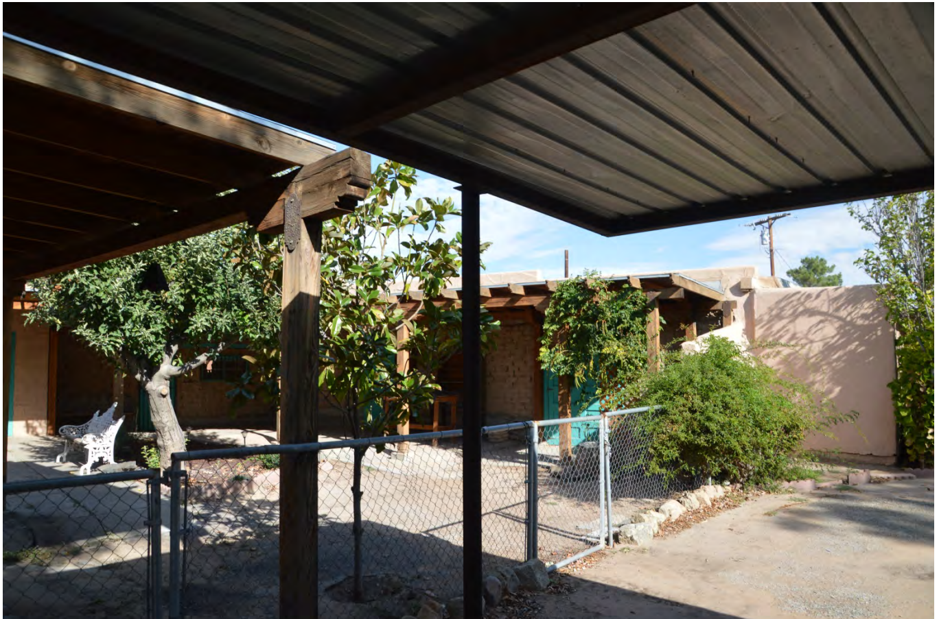
PHOTO OF REAR OF DWELLING FROM CARPORT THAT WAS REMOVED (Taken 10/19/17)
