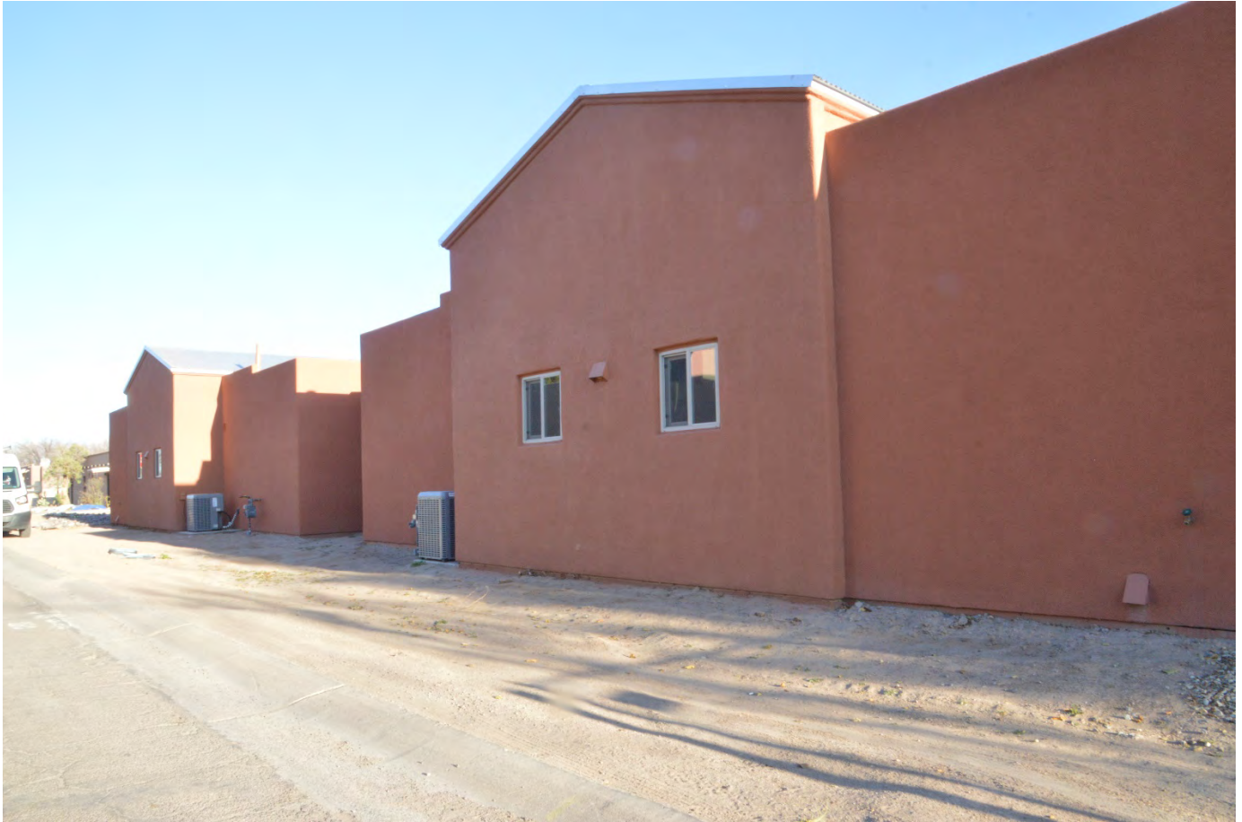
PHOTO OF THE PROPERTY FROM CALLE DE COLON
