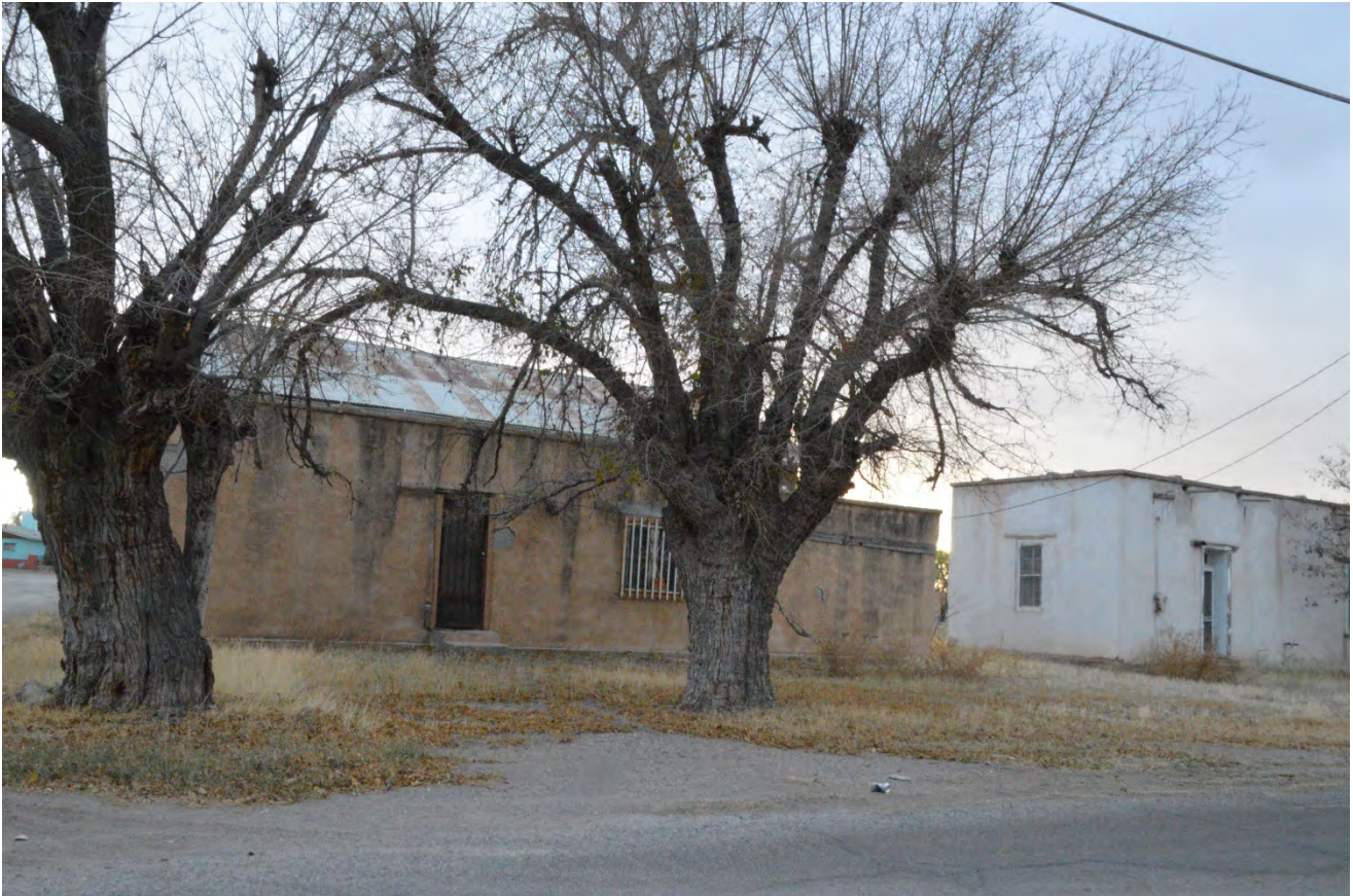
OLD STORAGE STRUCTURE IMMEDIATELY TO THE SOUTH
