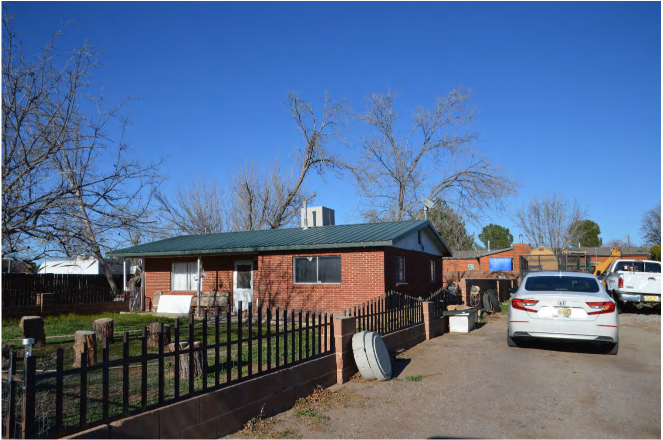
PHOTO OF THE DWELLING FROM CALLE DE GUADALUPE
