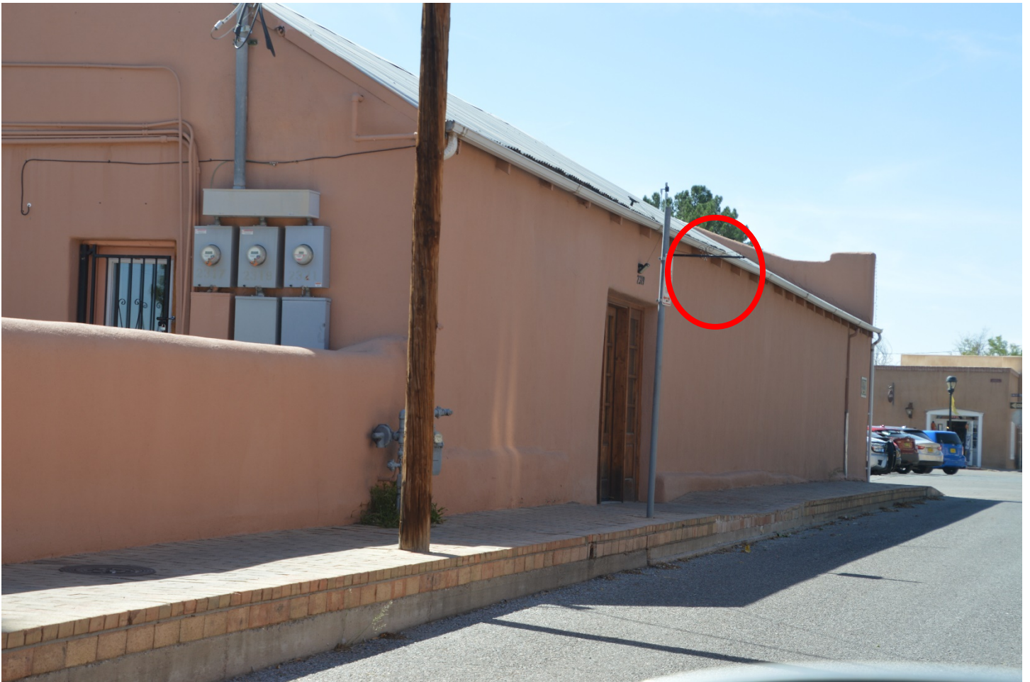
PHOTO FROM CALLE DE SANTIAGO SHOWING LOCATION OF SIGN
