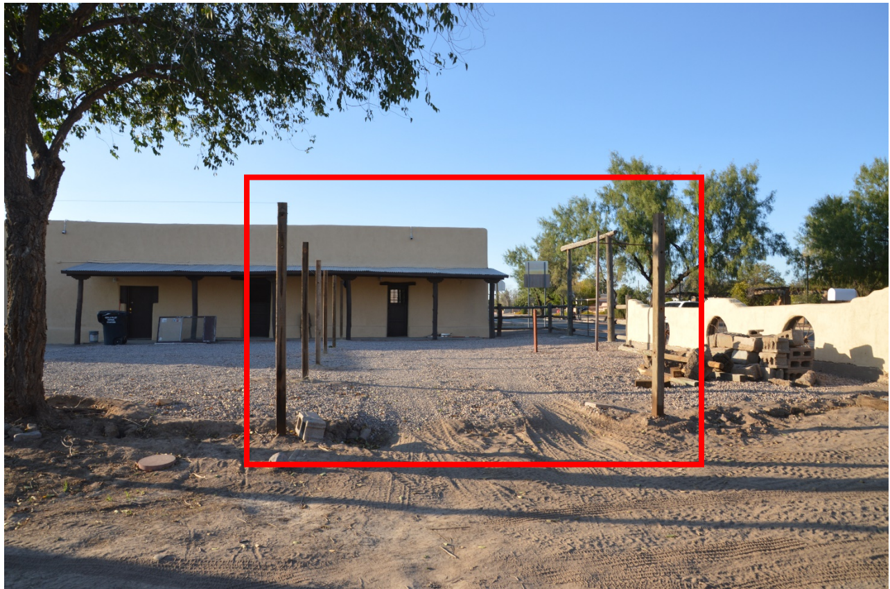
PHOTO FROM PROPERTY TO THE SOUTH SHOWING PROPOSED GATE LOCATION
