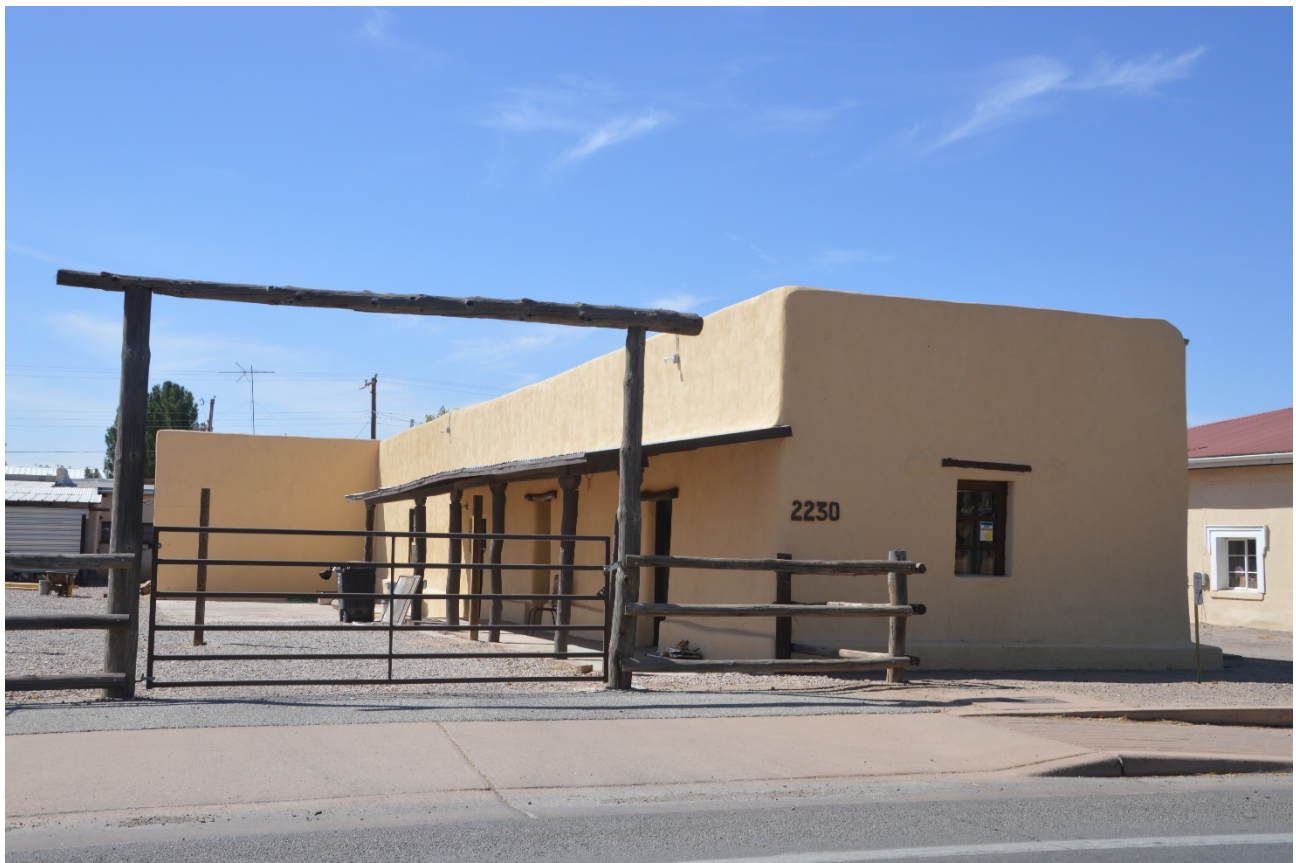
PHOTO FROM AVENIDA DE MESILLA SHOWING THE SUBJECT PROPERTY
