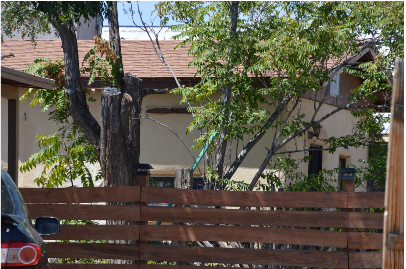
VIEW OF REAR OF DWELLING
