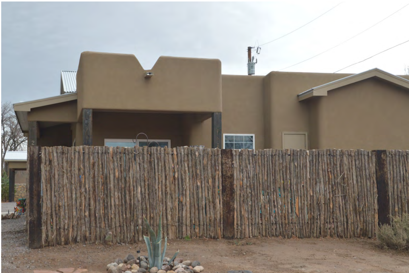
PHOTO OF SIMILAR FENCE AT FRONT OF 2219 CALLE DE PARIAN
