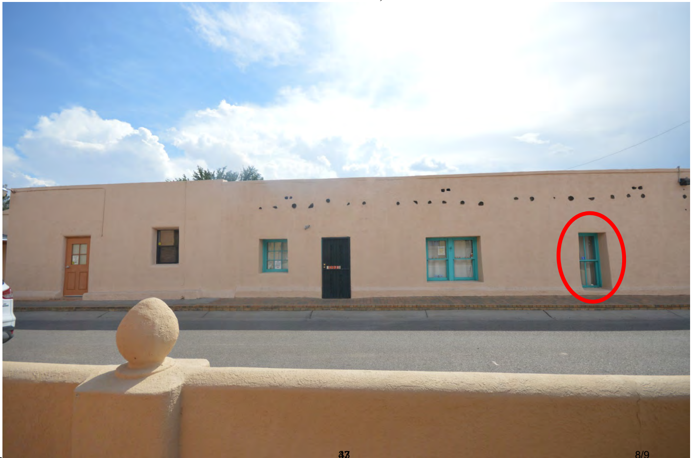
PHOTO OF WALL SHOWING OTHER DOORS, AND WINDOW TO BE REPLACED
