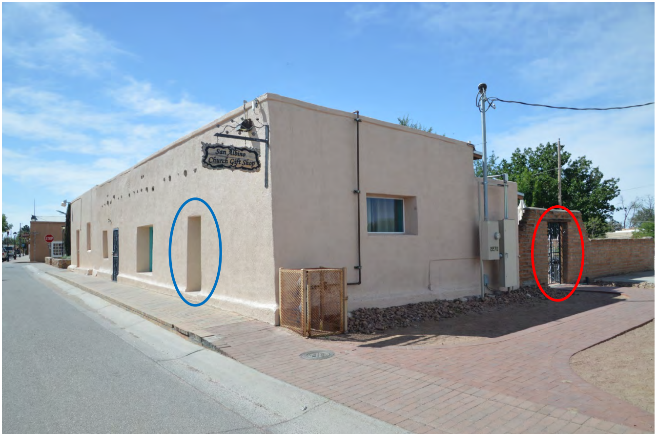
PHOTO OF FRONT OF STORE SHOWING CURRENT ENTRANCE AND PROPOSED ENTRANCES
