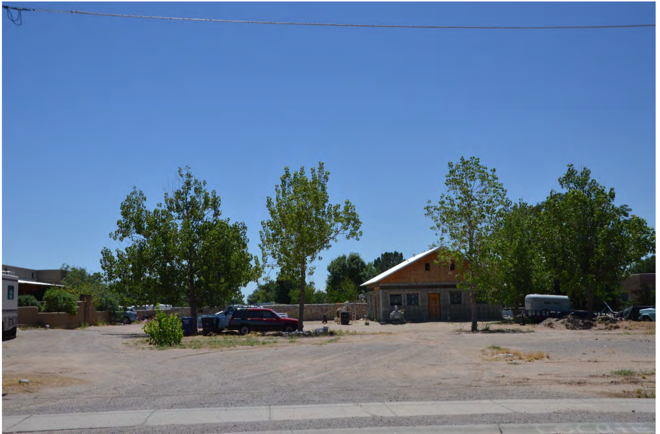
PHOTO OF THE DWELLING UNDER CONSTRUCTION AT 2230 ON CALLE DEL SUR
