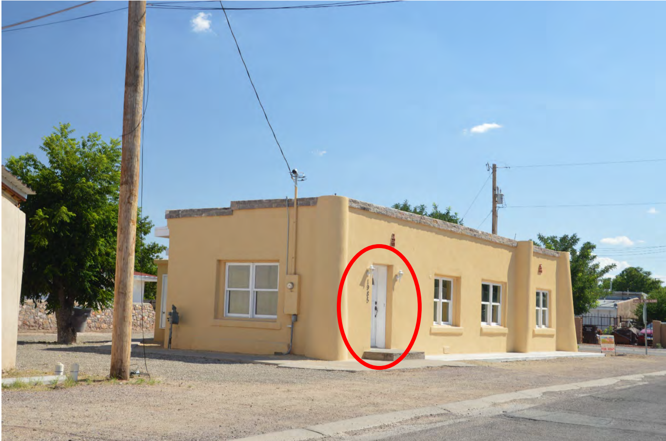
PHOTO FROM CALLE DE COLON SHOWING ONE OF THE EXIT DOORS
