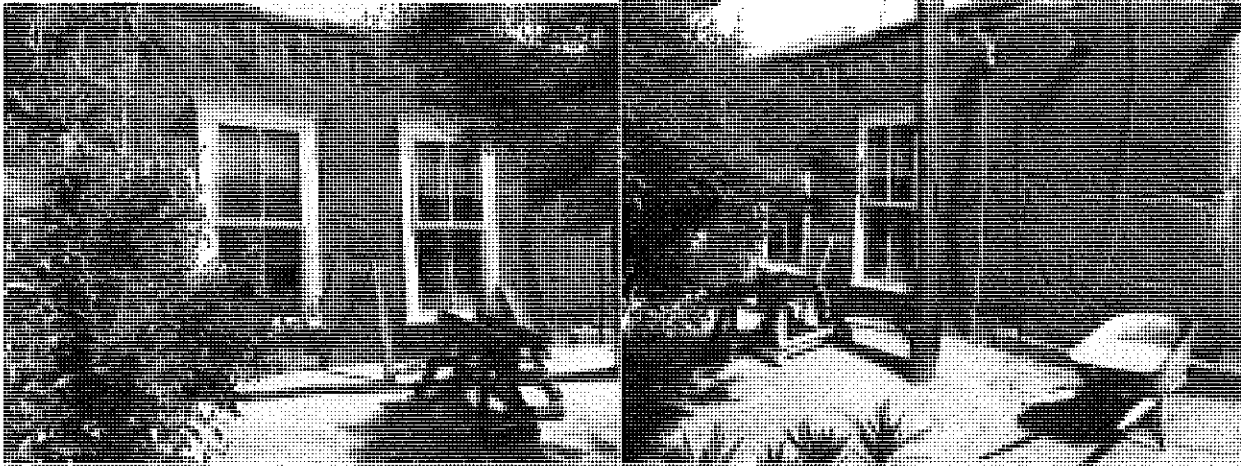
NW section of North Wall with mud plaster
