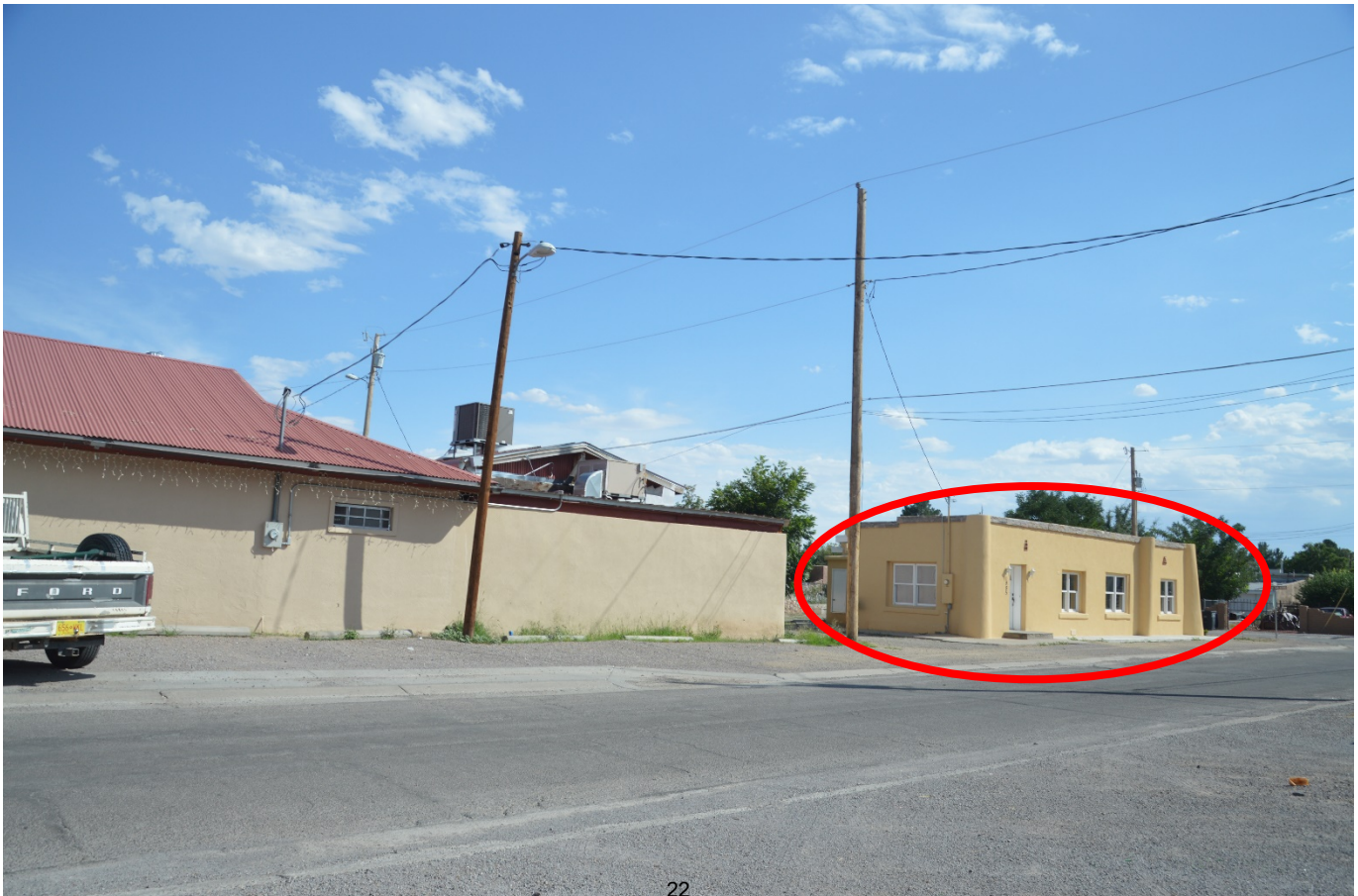
PHOTO OF THE PROPERTY FROM AVENIDA DE MESILLA SHOWING PROXIMITY TO PALACIOS BAR
