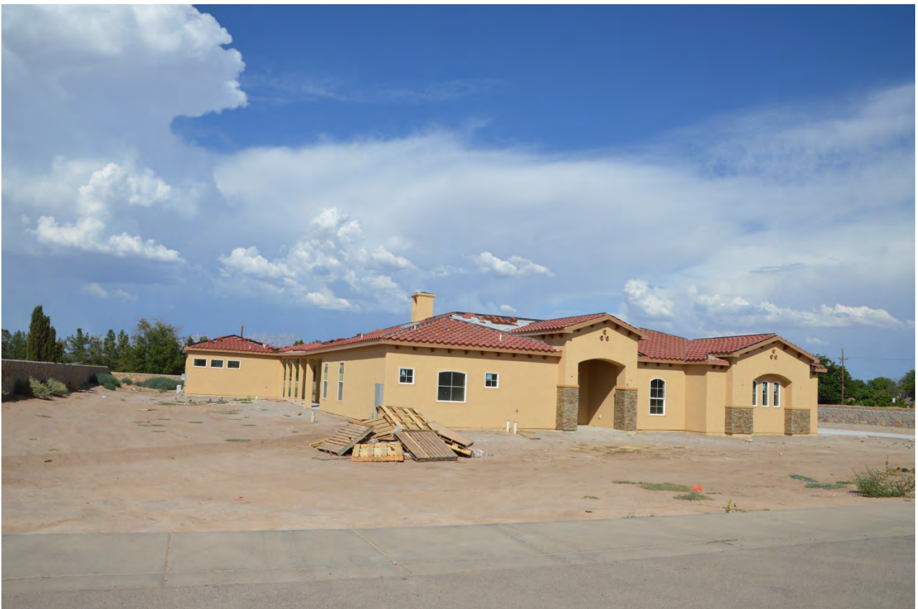
PHOTO OF NEIGHBORING DWELLING UNDER CONSTRUCTION TO THE NORTH
