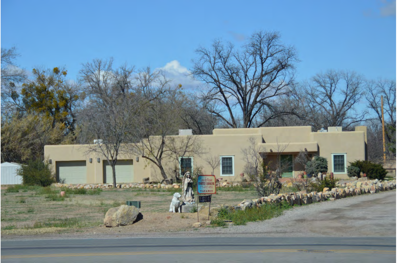
PHOTO OF THE DWELLING AT 2140 CALLE DEL NORTE
