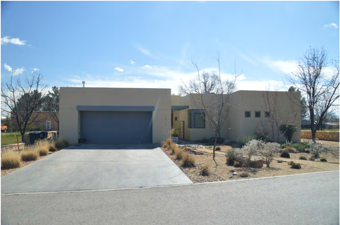
PHOTO OF THE DWELLING AT 1910 CALLE PACANA
