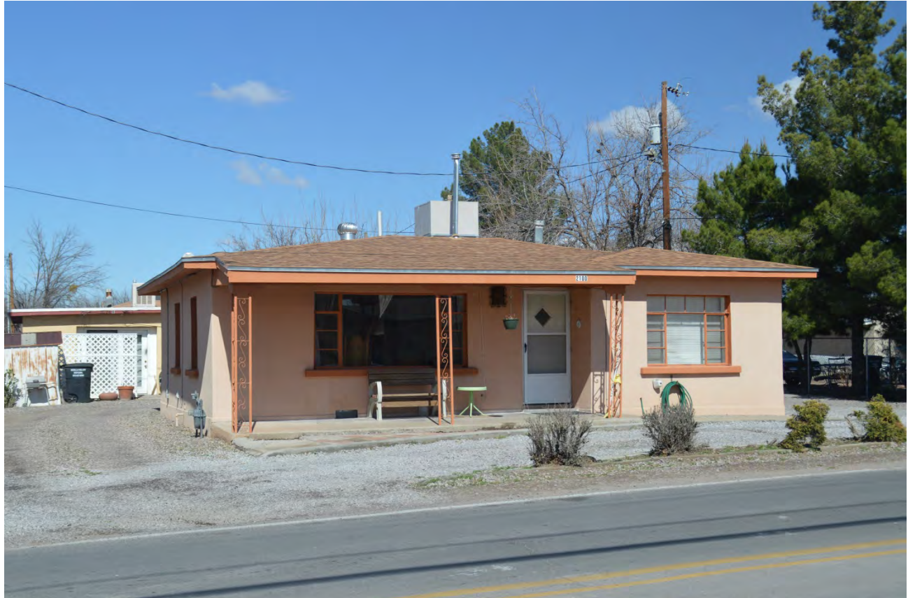
PHOTO OF THE DWELLING AT 2100 CALLE DEL NORTE
