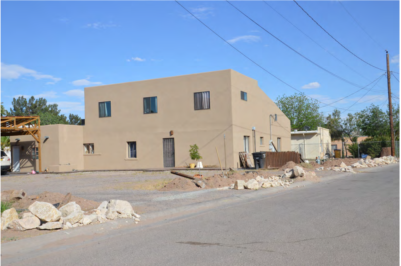
PHOTO OF FRONT OF PROPERTY FROM CALLE TERCERA
