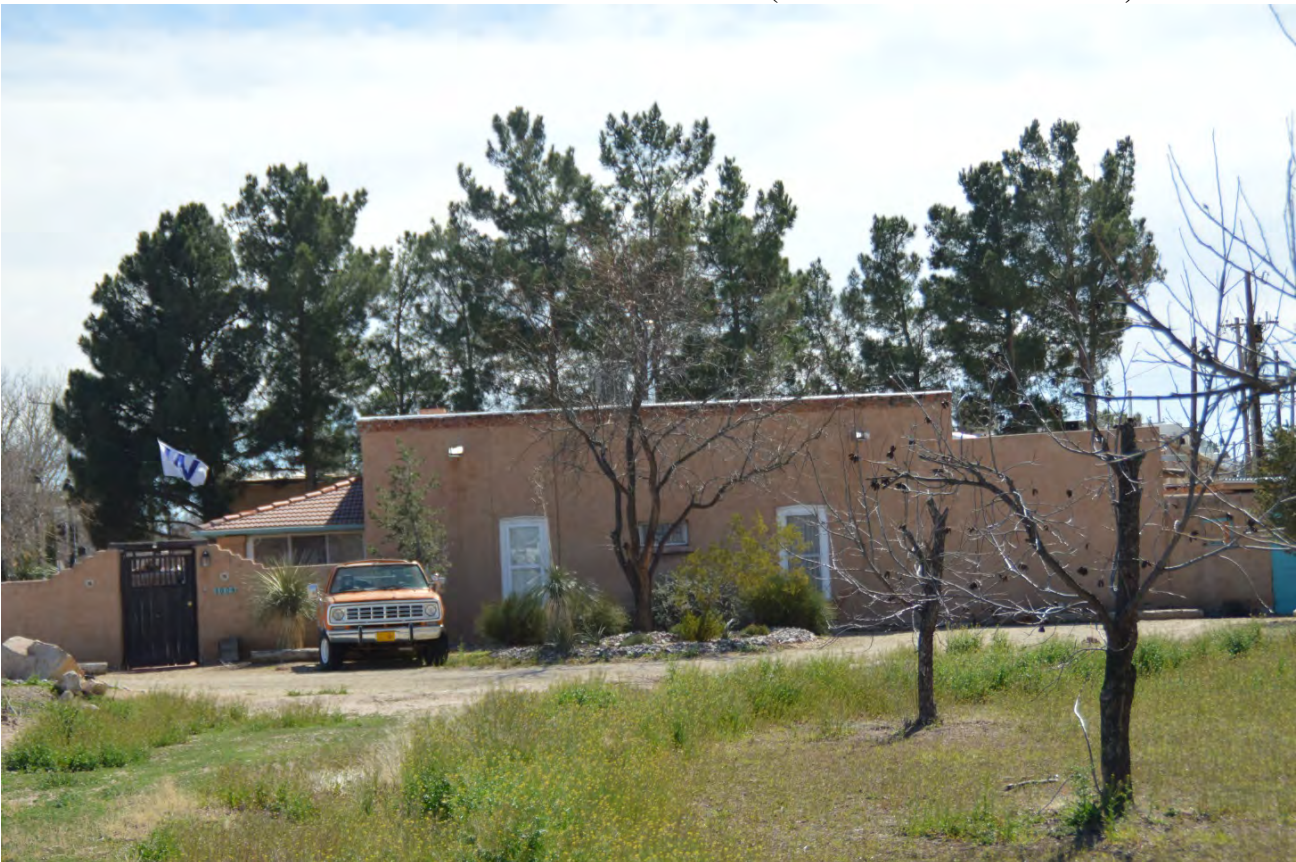
PHOTO OF THE DWELLING TO THE EAST (2008 CALLE DE EL PASO)
