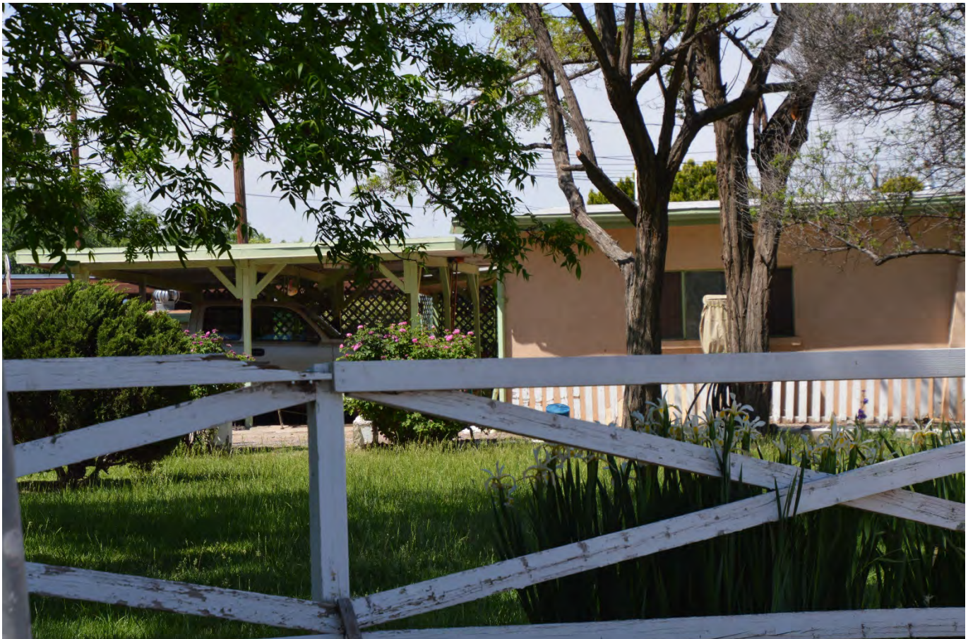
PHOTO OF THE STRUCTURE FROM CALLE DEL NORTE
