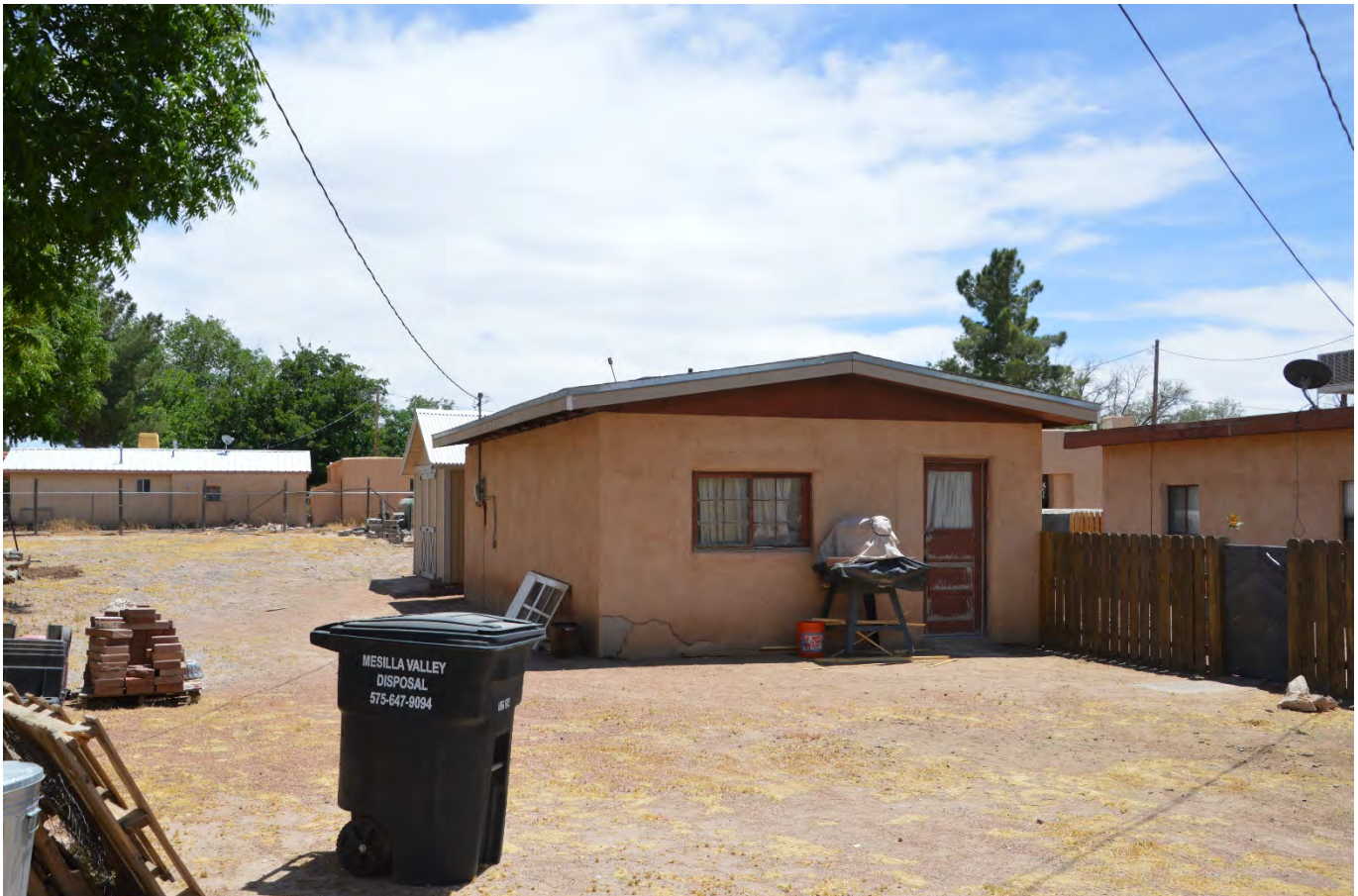
PHOTO OF THE STRUCTURE FROM CALLE DE PARIAN
