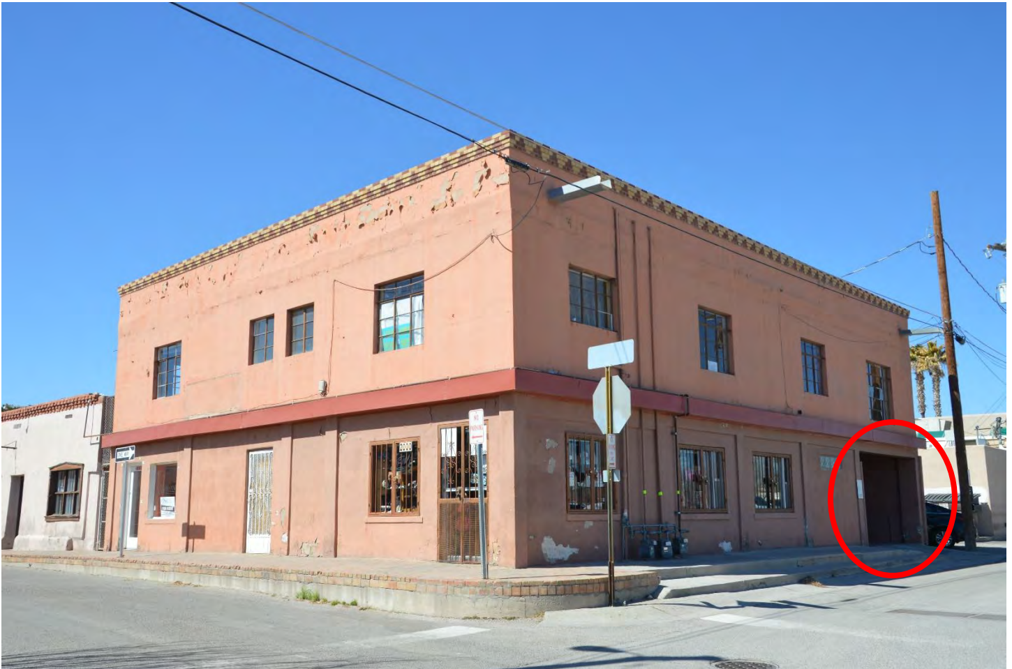
PHOTO OF THE STRUCTURE FROM CALLE DE SAN ALBINO SHOWING OPEN GARAGE AT FAR RIGHT
