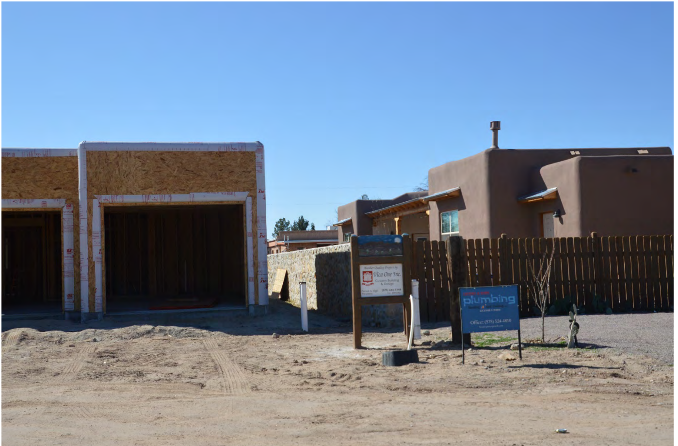
PHOTO OF THE NEIGHBORING DWELLING AND ROCK WALL
