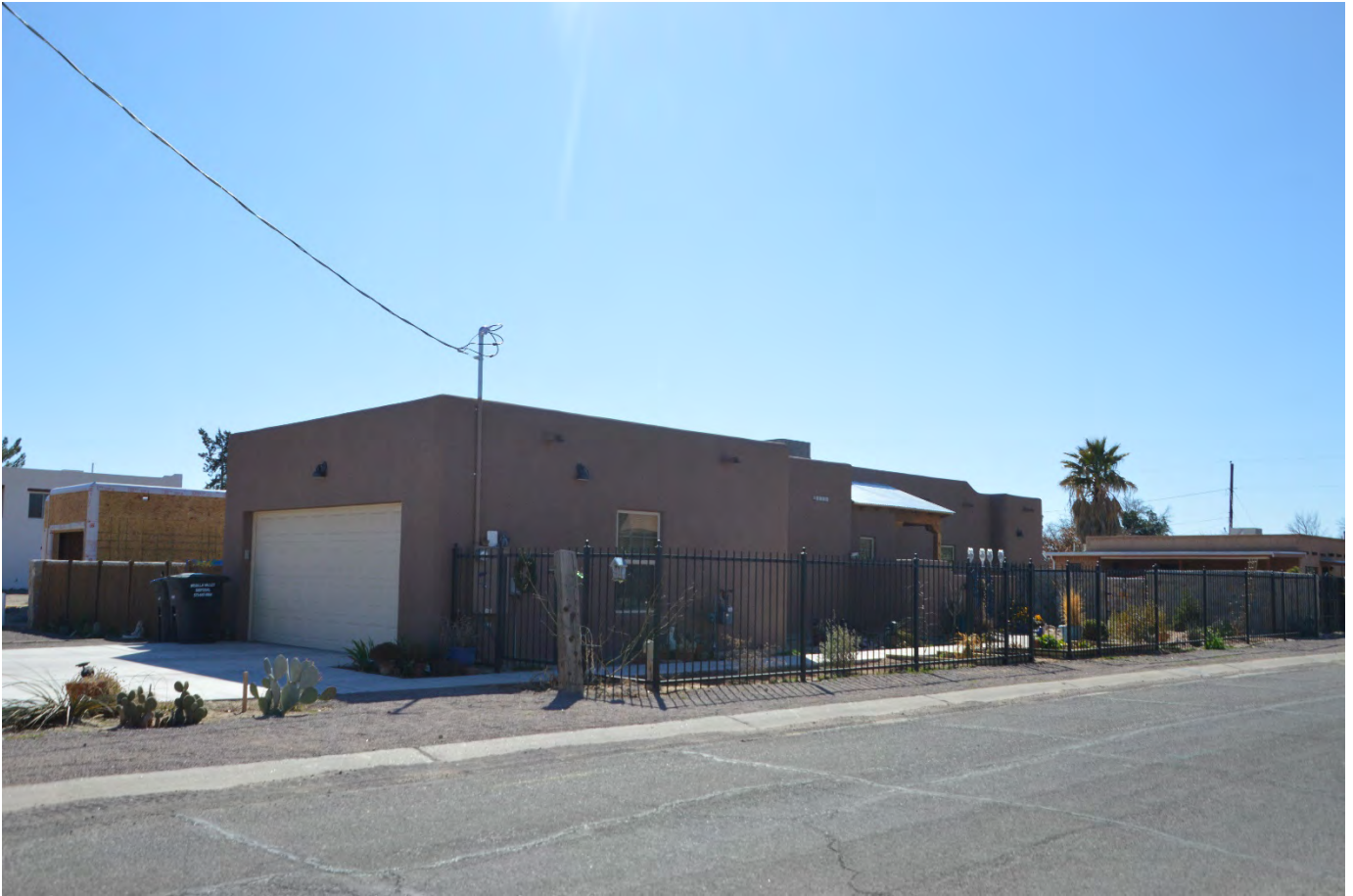
PHOTO OF THE SUBJECT DWELLING FROM CALLE DE COLON
