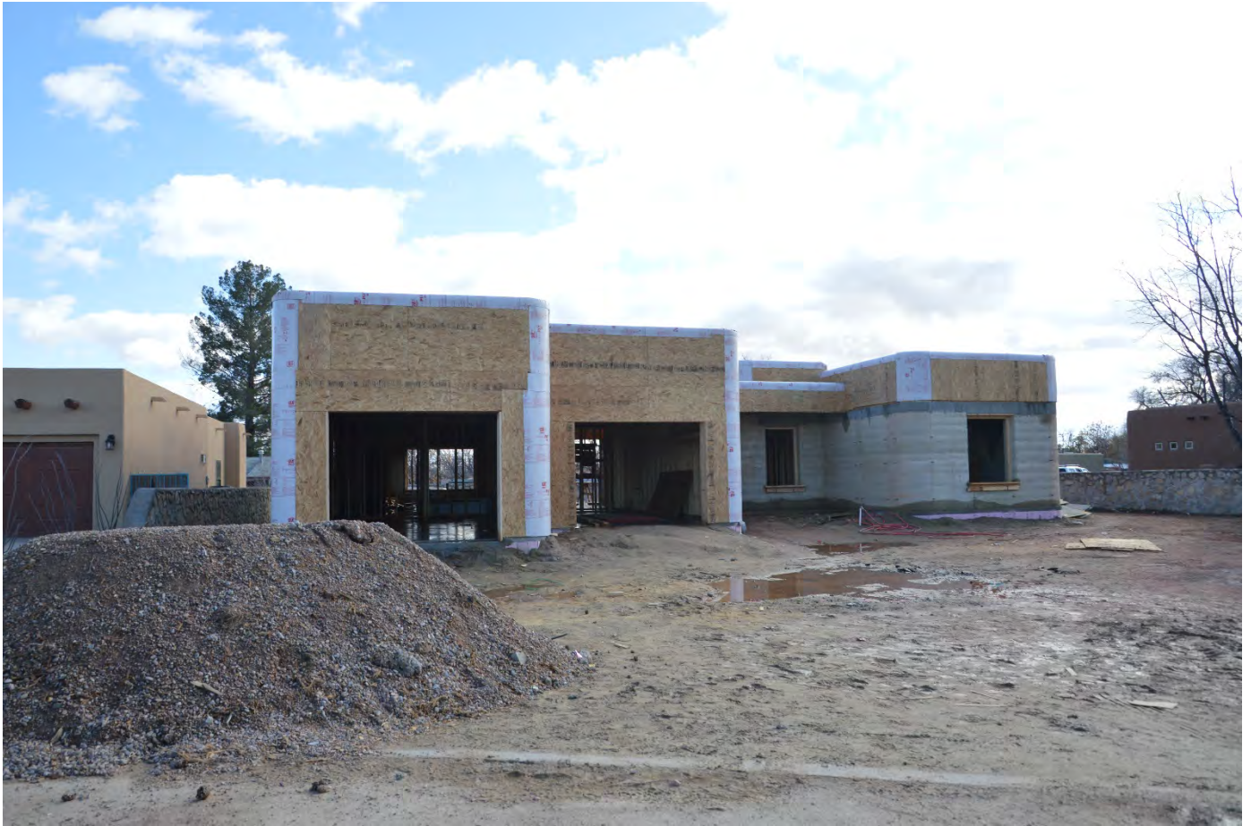
PHOTO OF THE PROPERTY WITH DWELLING UNDER CONSTRUCTION
