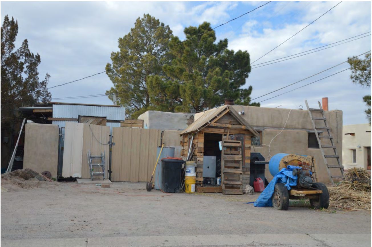
PHOTO OF SOUTH SIDE OF PROPERTY FROM CALLE DE COLON SHOWING SHED AND AREA TO BE FENCED (PHOTO USED IN CITATION)
