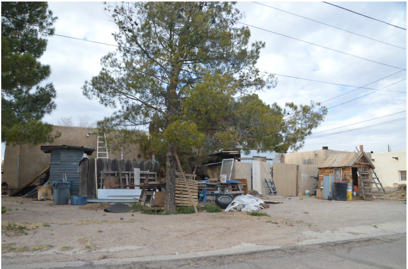
PHOTO OF OTHER CODE ISSUES ON THE PROPERTY RESULTING IN CITATION (IN PROCESS OF BEING ADDRESSED)
