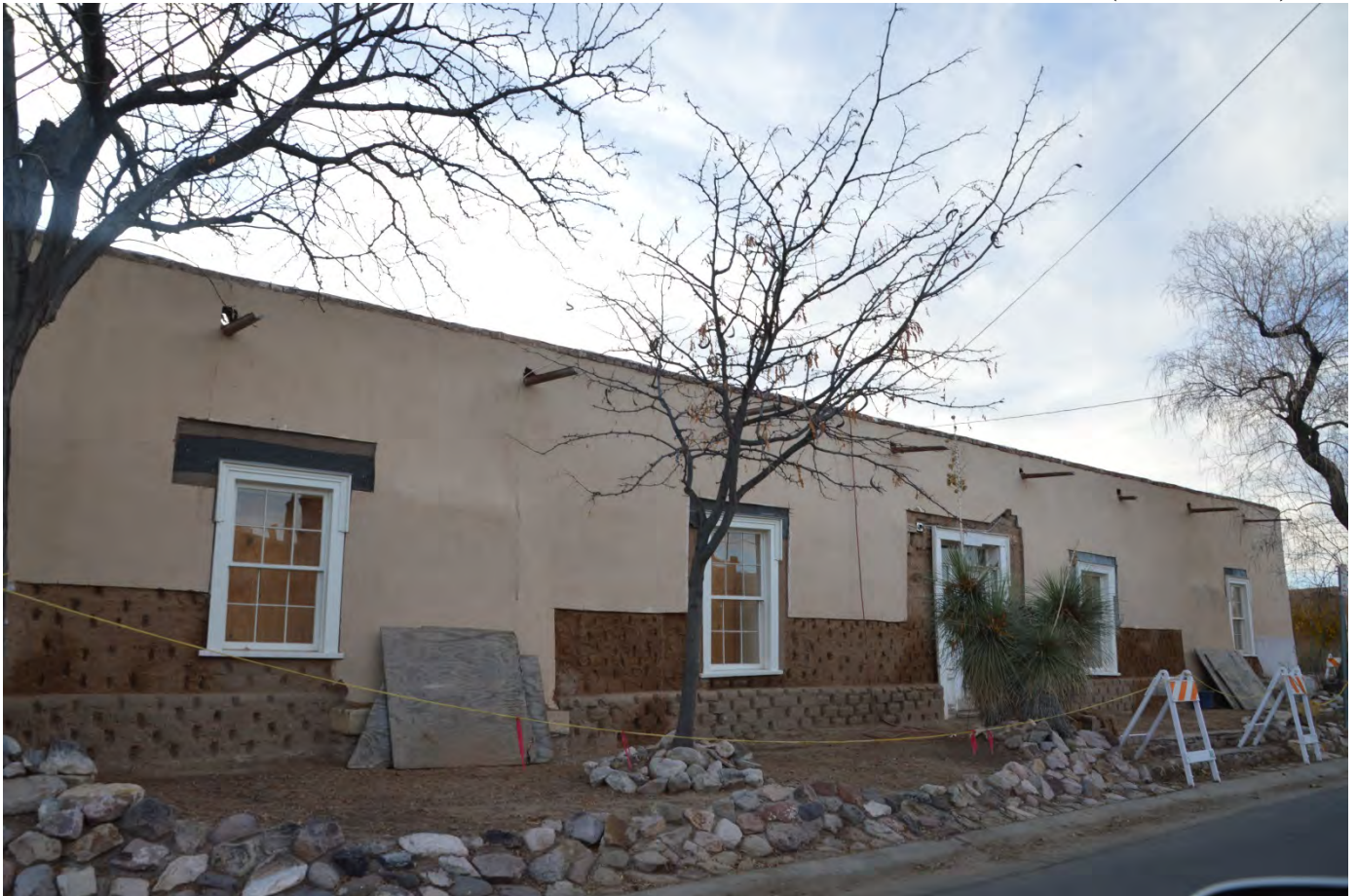
PHOTO OF THE SUBJECT STRUCTURE FROM CALL DE GUADALUPE (EAST SIDE)
