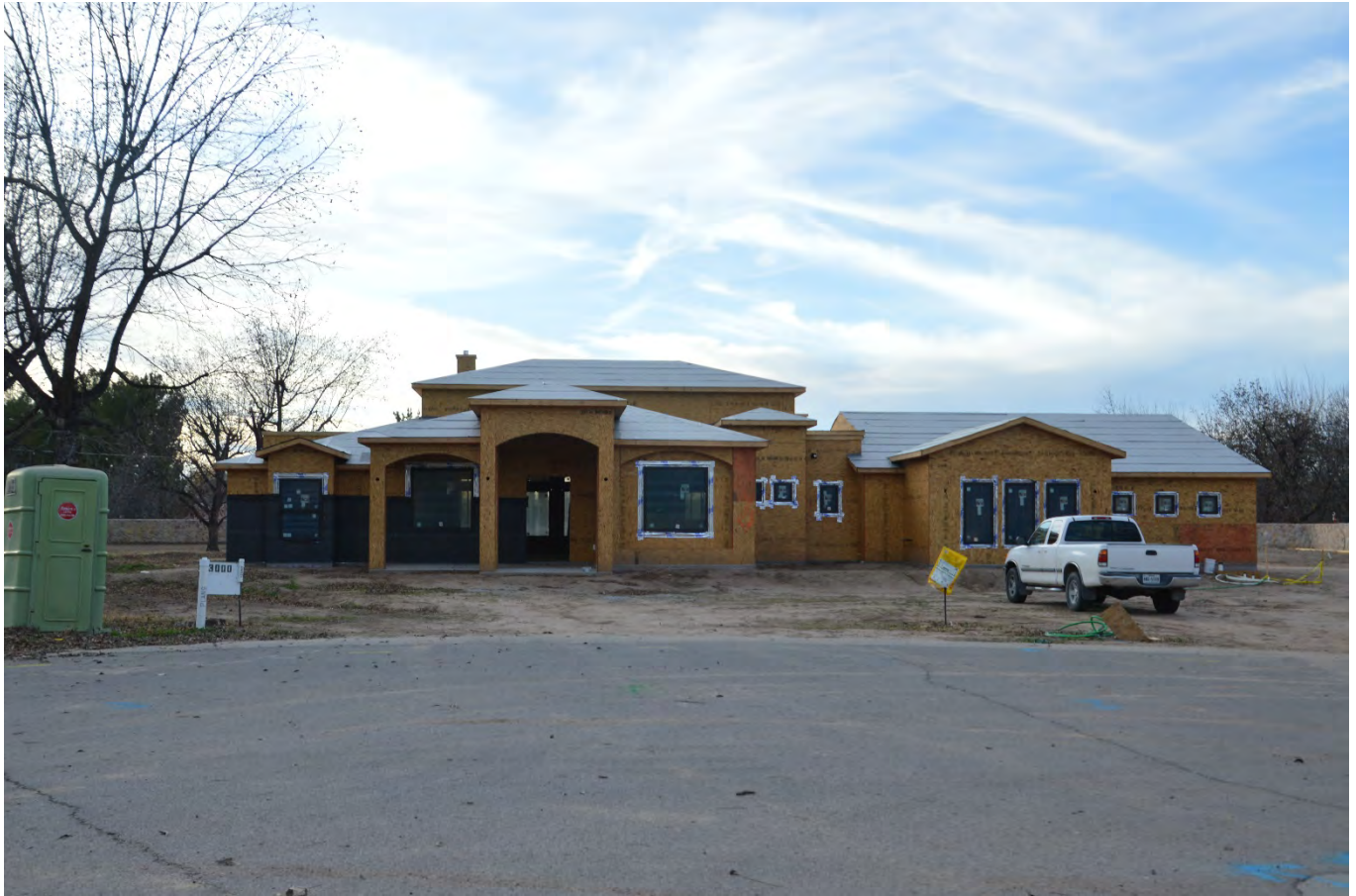
PHOTO OF PROPERTY FROM MESILLA VERDE TERRACE
