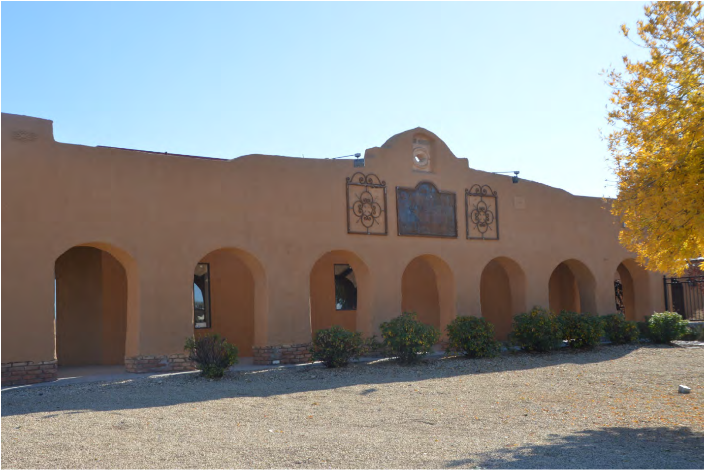
PHOTO FROM CALLE DE MERCADO SHOWING SIGN LOCATION
